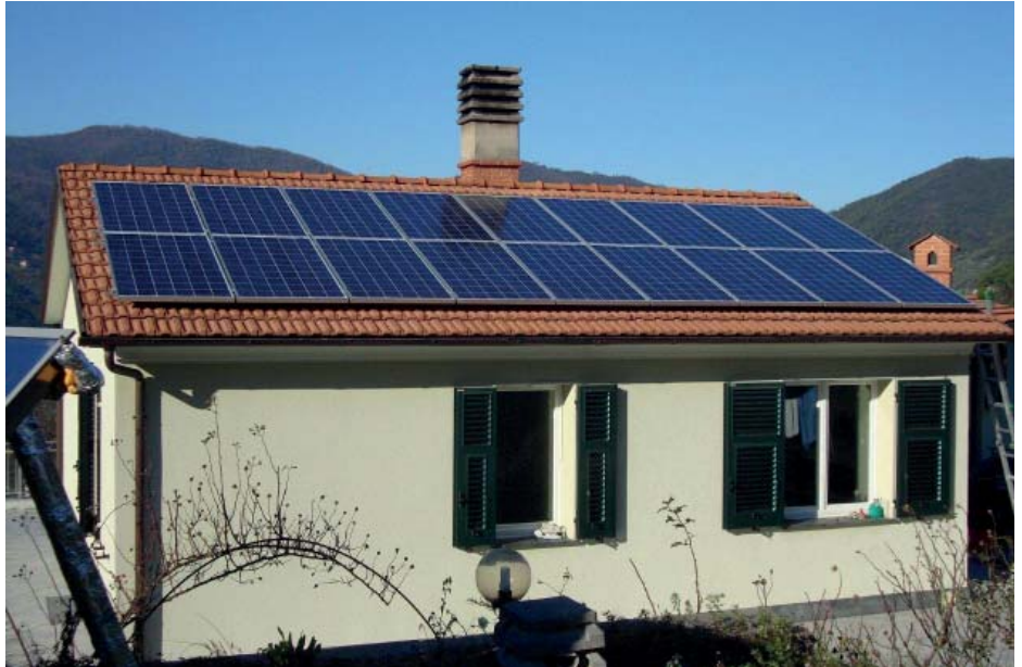
Photovoltaic plant on retail business
