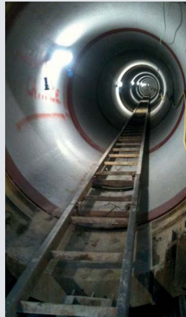
Cosoletto - tunnel under construction
