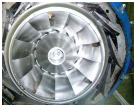
O&M - Francis turbine dismantling for checking and cleaning
