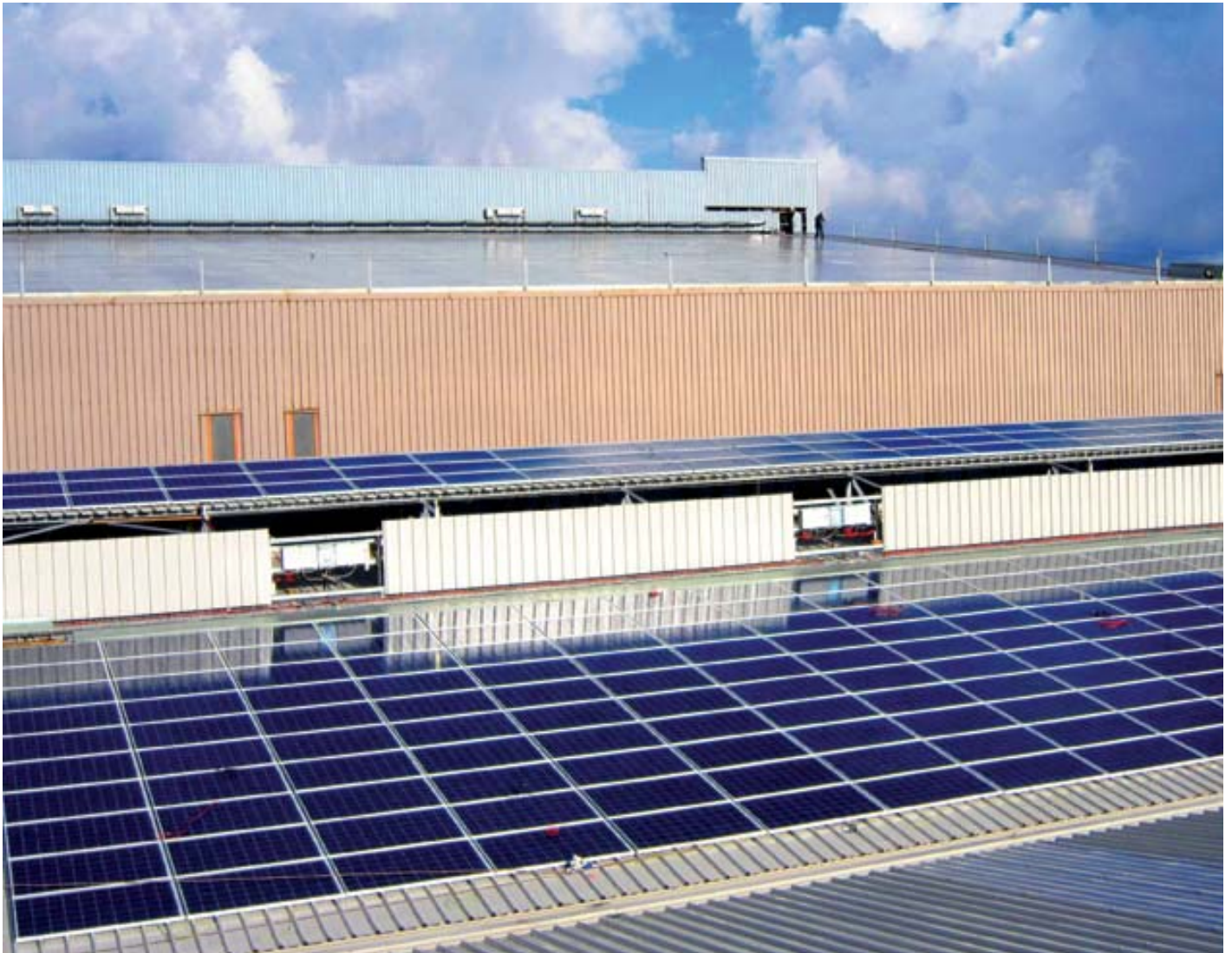
Duferco photovoltaic plant of 4.869 kWp Giammoro (Sicily)
