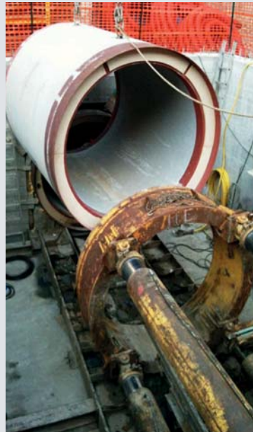
Cosoletto tunnel - Pusher station
